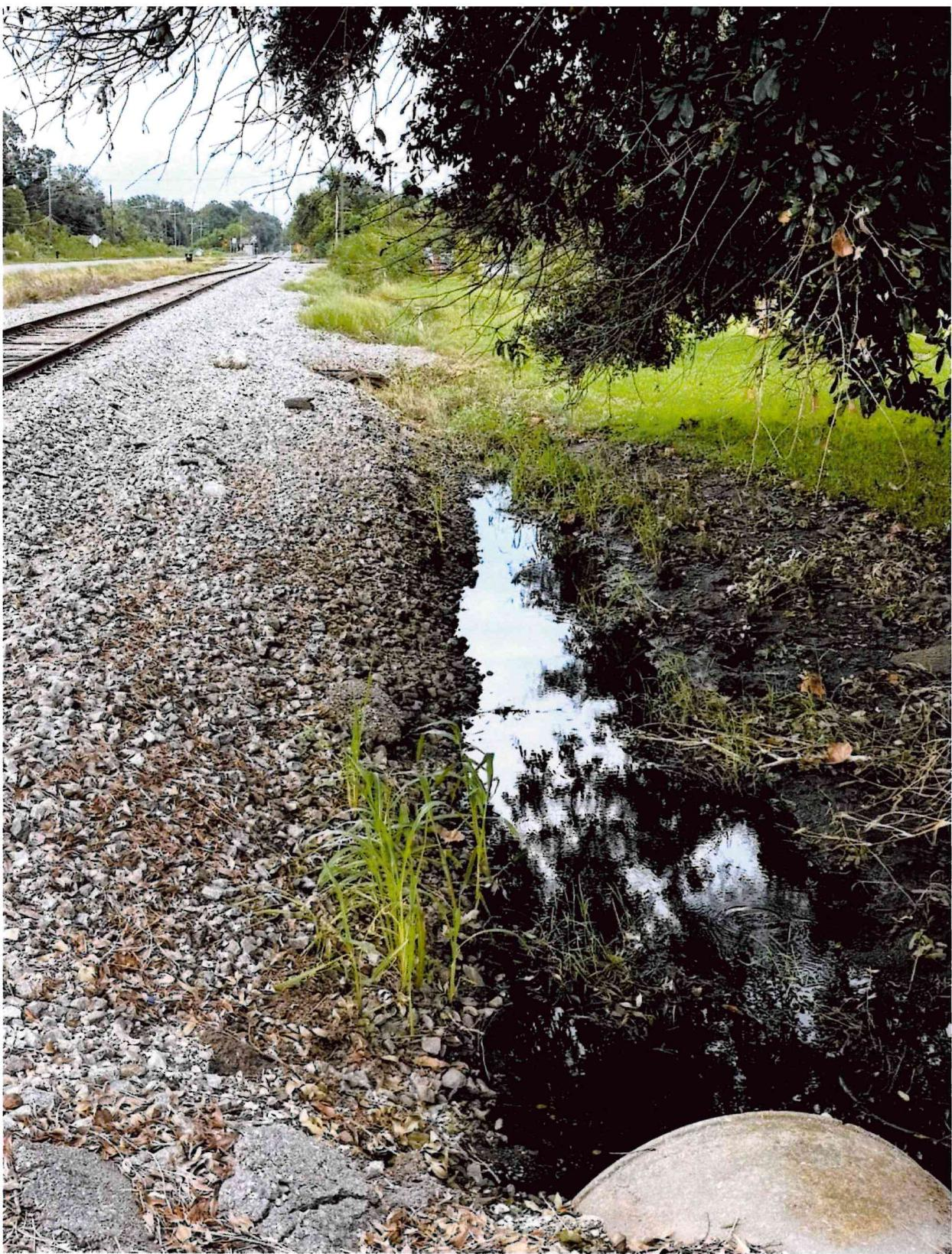
**This picture shows the embankment falling into the ditch, obstructing the flow of water.**
