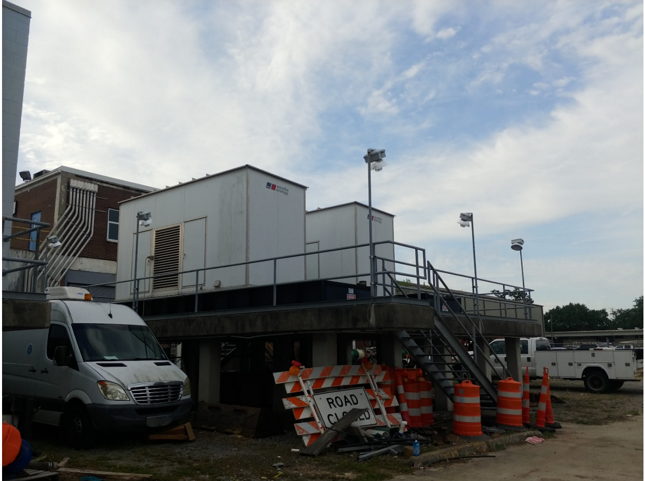
Two generators elevated on platform with 3,000 gallon belly tanks
