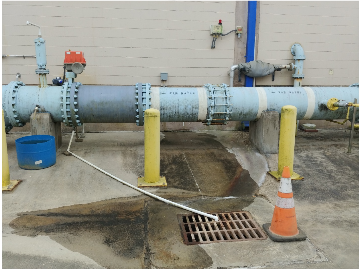
Storm drain with potable water bleed off drain off
