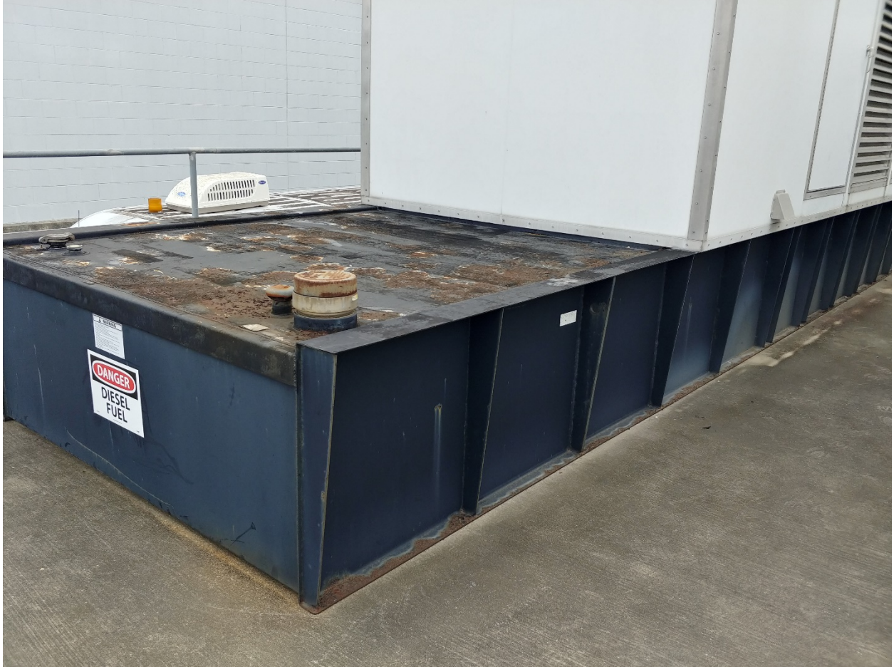
3,000 gallon double-walled belly tank for generator
