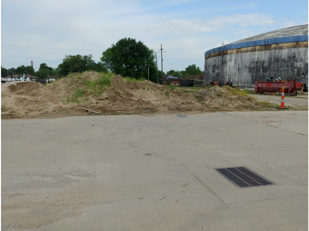
Uncontained fill piles for construction project were present. Photo shows relationship to storm drain
