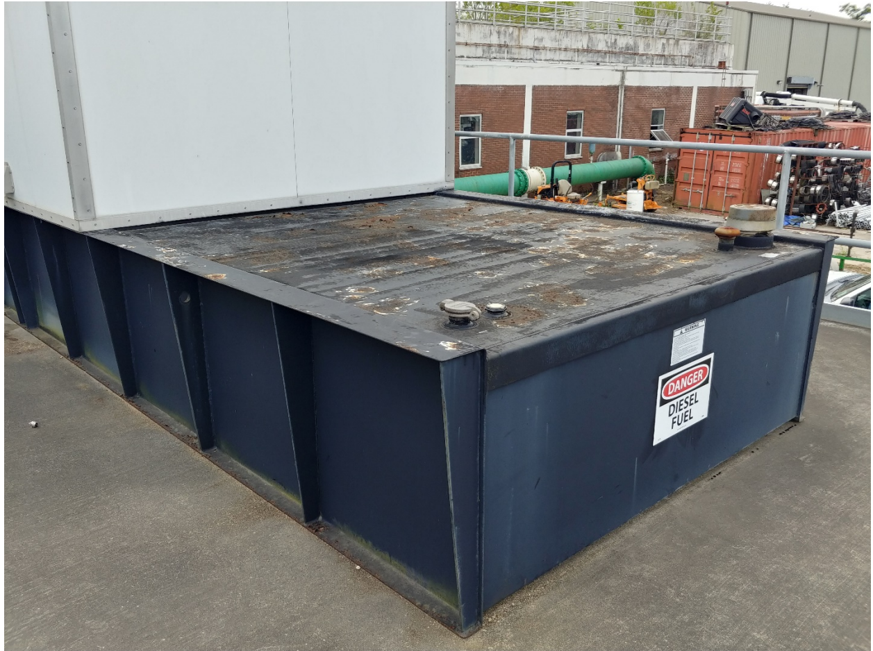
3,000 gallon double-walled belly tank for generator
